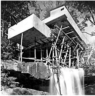
Scaffolding (©F.L.Wright Fdn.)
