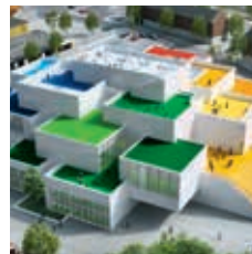
The surfaces of the colored terraces are made of leftover materials from sneaker production by several different international sports brands.
