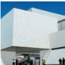
The building is covered with white facing bricks with a size of 7 x 23.5 in. (18 x 60 cm), giving the illusion that the building is made of LEGO® bricks.
